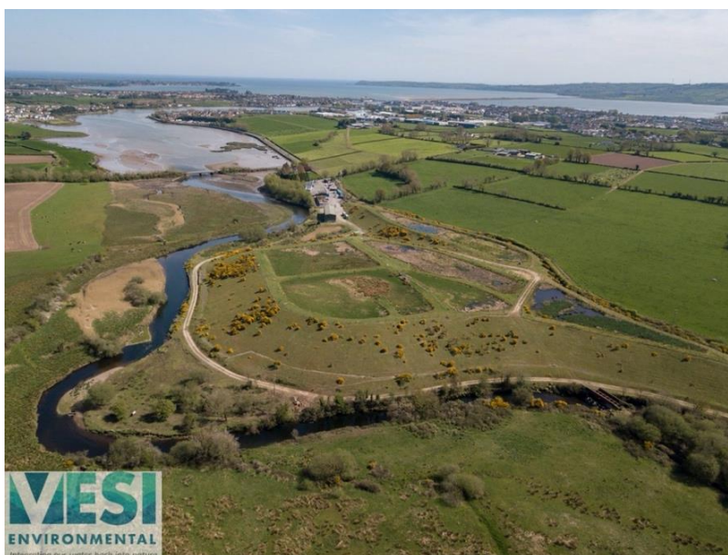
Figure 4. Dungarvan Landfill catering for landfill leachate since 2007, Co. Waterford.
